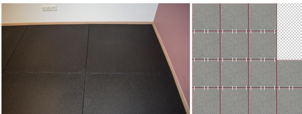
Press tiles together; installation of tiles in a chessboard formation
