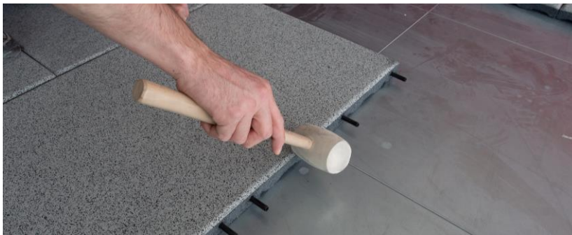
Closing the gaps with a hammer
