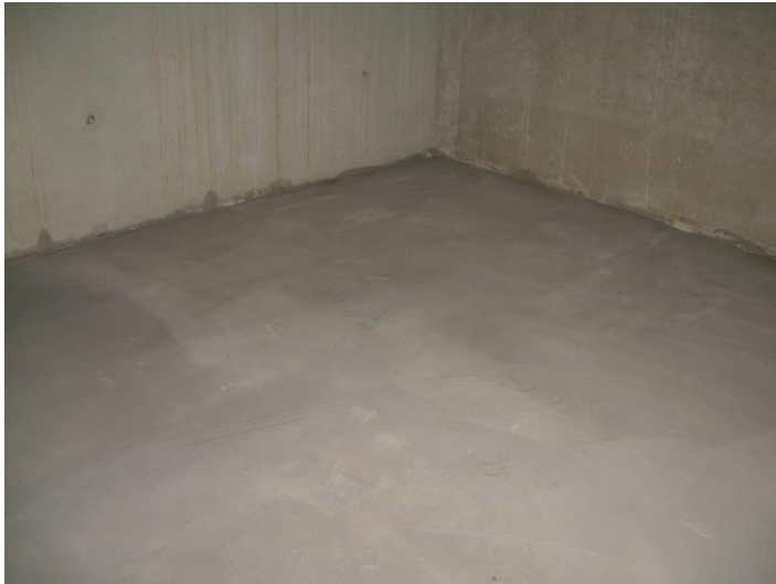
Even, suitable substrate made of poured screed
